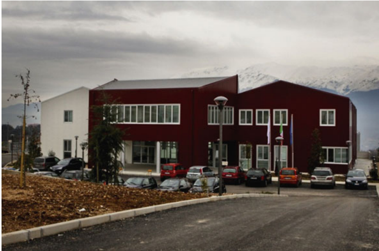
Fig. 19.21 The new prefabricated music conservatory of L'Aquila
