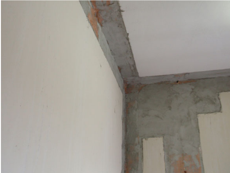
Fig. 19.19 Improvement of connections of infilled masonry panels with the R/C structure, against tilting
