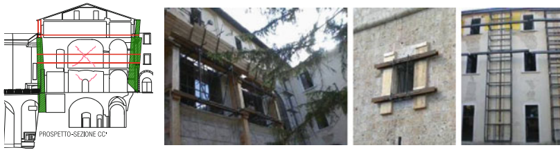
Fig. 20.17 Provisional interventions: connection of the internal and external façades
