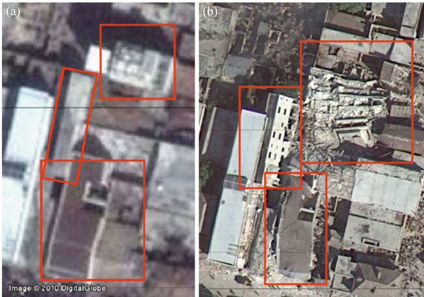
Fig. 9.6 Haiti earthquake 2010: a satellite image prior to event; b a satellite image after the event (Courtesy EERI, 2010, World Bank)
