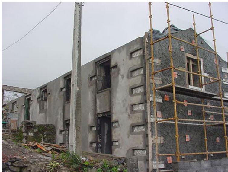
Fig. 9.2 Wire mesh in plaster covering
