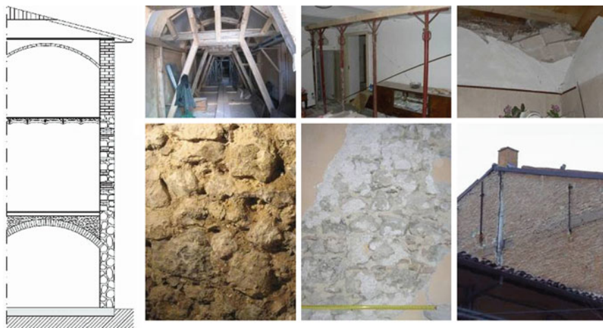
Fig. 20.25 Vertical cross section of the building in Piazza della Prefettura ( left ); types of floors: stone vaults, steel beams and brick elements, vaults made of sailor brick masonry; types of masonry: irregular stone, stone with brick courses, brick masonry
