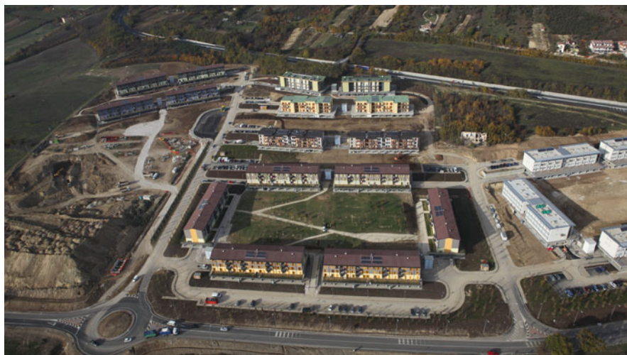
Fig. 19.13 Aerial view of one settlement of the Project C.A.S.E. (Bazzano) on October 29, 2009. Twenty-one buildings are all completed and inhabited by about 1,600 people
