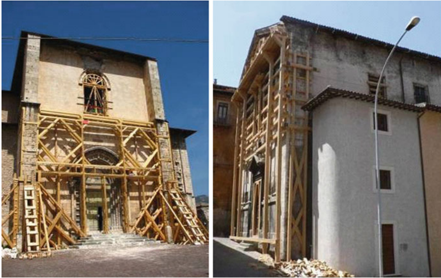
Fig. 20.8 Intervention during works at S. Domenico's church and concluded intervention at Evangelica's church in the historical centre of L'Aquila
