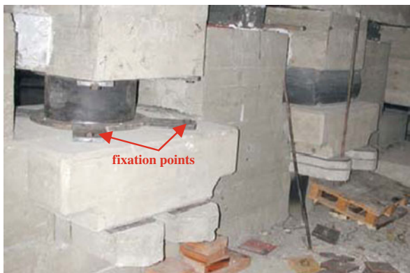
Fig. 17.25 Installed new and old bearing
