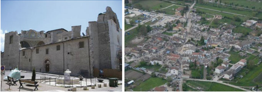
Fig. 20.1 Santa Maria di Paganica's church in the historical centre of L'Aquila ( left ). Aerial view of the destroyed Onna village ( right )
