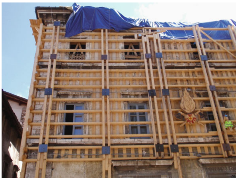
Fig. 19.22 Provisional works on a building of the historical centre of L'Aquila
