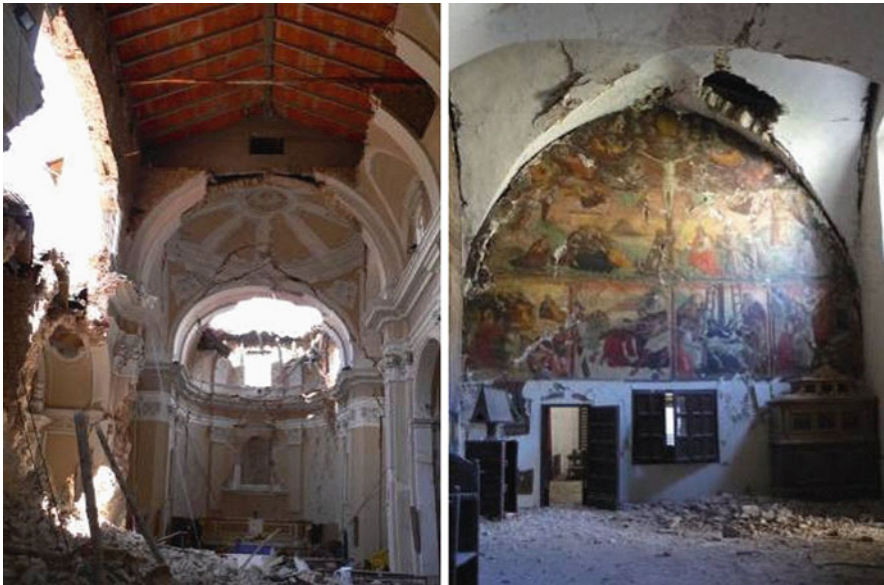
Fig. 20.4 Inside view of San Marco's church ( left ) and of Beata Antonia's church ( right ) in the historical centre of L'Aquila: in the Beata Antonia's church the Fire Brigade provisional interventions repositioned the removed tie rods
