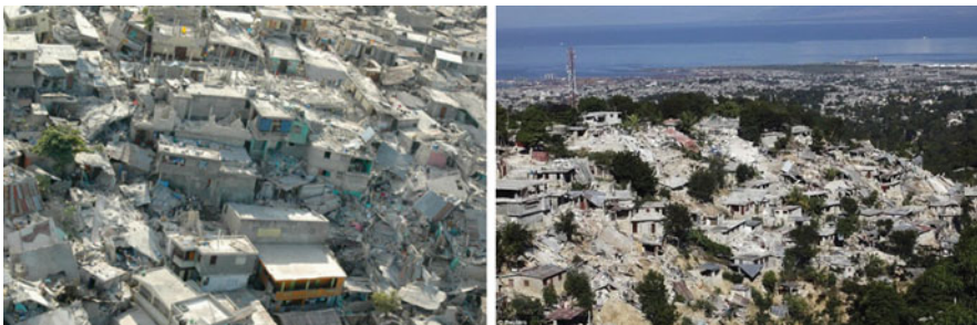
Fig. 9.8 Haiti earthquake. Overview of damage caused to buildings (photos: http://www.refinery29.com/pipeline/img/earthquake-haiti.jpg and http://3.bp.blogspot.com/_U54NM9QE5VY/S07Fcu30qDI/AAAAAAAAAJY4/p06ii_gUrbl/s640/haiti+earthquake.jpg )
