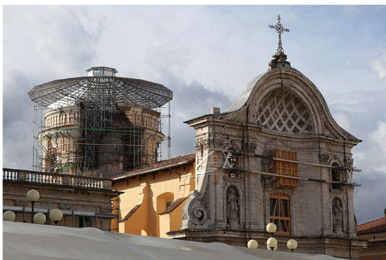
Fig. 19.23 Provisional works in the church of Anime Sante in L'Aquila
