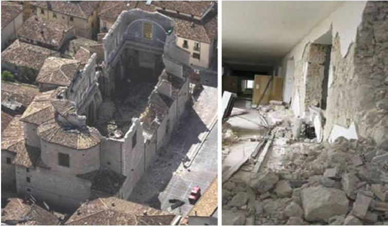
Fig. 19.12 The partial collapses of S. Maria di Paganica and of the Abruzzi Museum in L'Aquila
