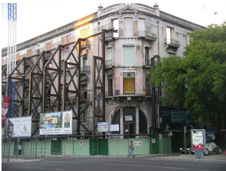
Fig. 9.1 Standing façade after the demolition of an interior core
