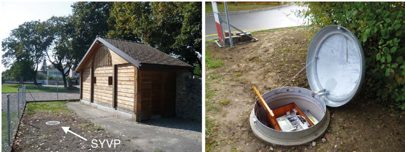
Figure 2. Alternative housing of the stations installed within the SSMNet renewal project. Left: small vault containing the sensor only and hut hosting the cabinet with the digitizer and communication instruments (station SYVP). Right: large vault containing the whole station (station SEPFL). The color version of this figure is available only in the electronic edition.
